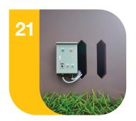
If you use gardening tools, make sure that the outdoor sockets are covered and that they operate via an earth leakage current breaker.
