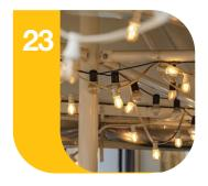
Don't use metal constructions such as vine supports or drying racks for outdoor lighting.
